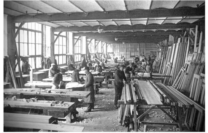
Figure 6. Traditional joinery in the workshop on the first floor of the Louis De Waele factory building (A3), designed by Henri Beyaert in 1888 (photo ca. 1900, CBRS CA).
